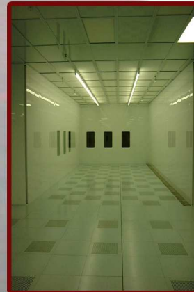
ISO4 Class cleanroom for electronic and microelectronic
